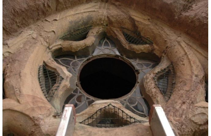
Fig 2: A medieval wrought iron frame supports the roundel
